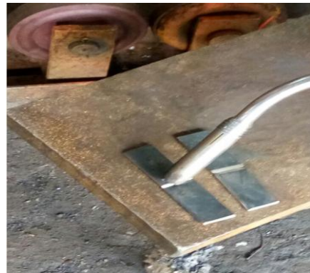
Welding on pieces
